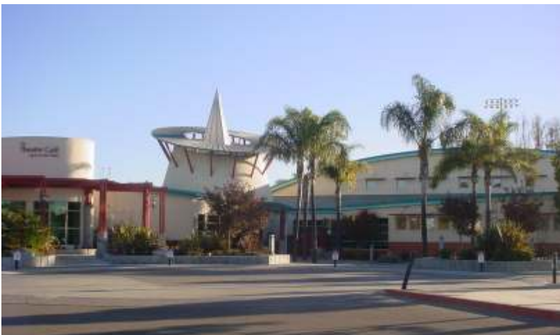
Innovative and widely recognized for its superior architecture, the Abel Maldonado Community Youth Center is a state-of-the-art facility that demonstrates Santa Maria's investment in its youth.
