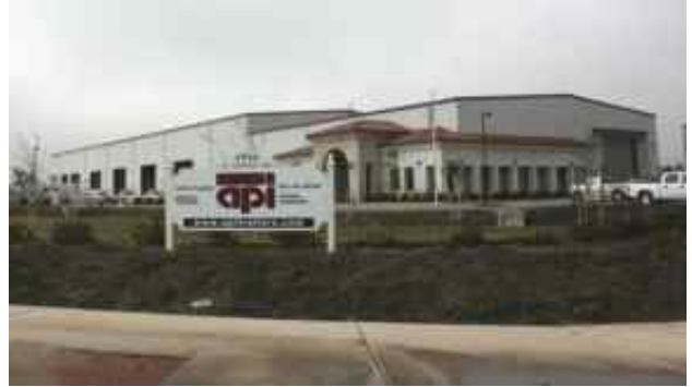
API (Atlas Performance Industries) manufacturing facility, located at 1916 West Stowell Road, Santa Maria
